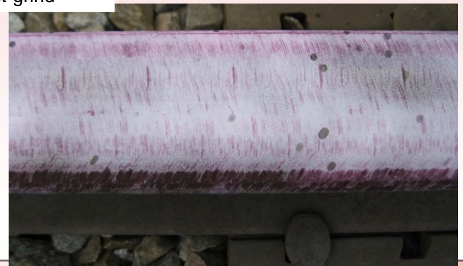
Rail photos are post-grind
