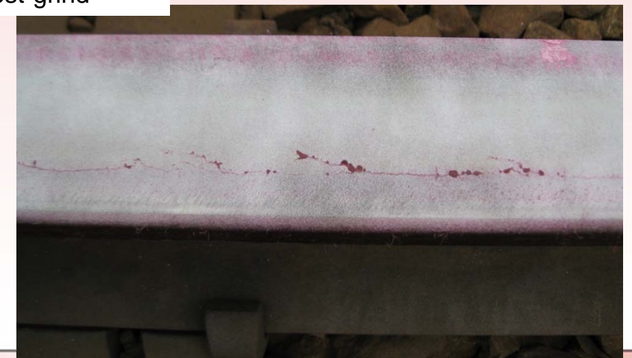
Rail photos are post-grind
